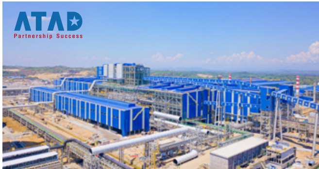
PROJECT NAME: HOA PHAT - DUNG QUAT STEEL PRODUCTION COMPLEX
