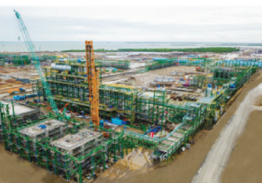
Long Son Petrochemical Complex
