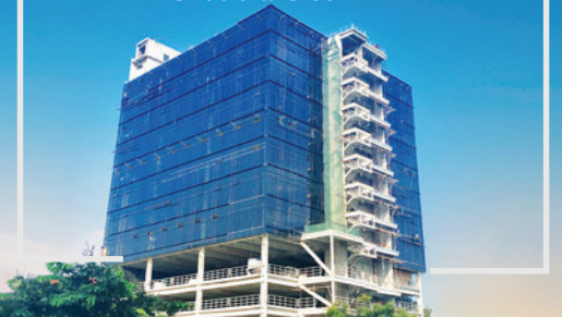
High-rise Building, Philippines
