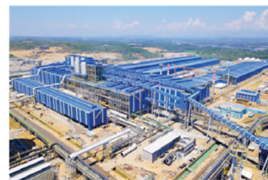
Hoa Phat - Dung Quat Steel Production Complex
